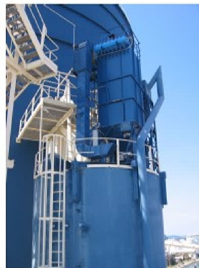
Dust collector FVL 3,0-64-78 Capacity 5.000 m 3 /h
