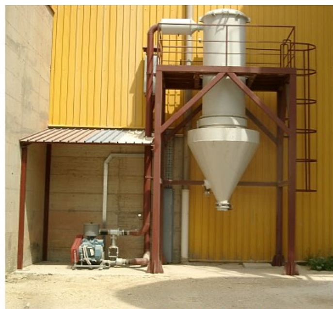
Vacuum cleaner VC-800 Capacity 800 m 3 /h
