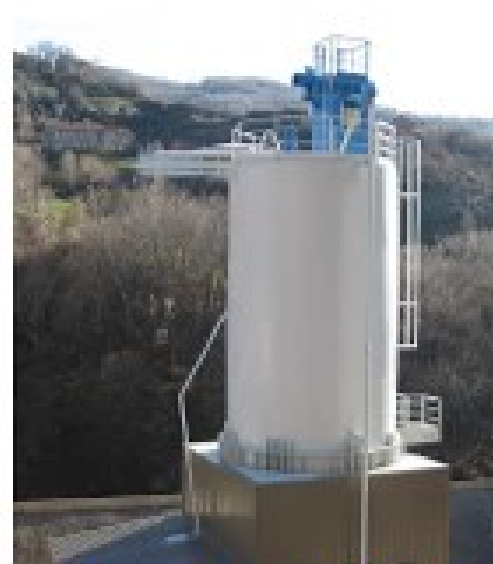
Dust collector FVS 2,0-36-29 Capacity 2.500 m 3 /h
